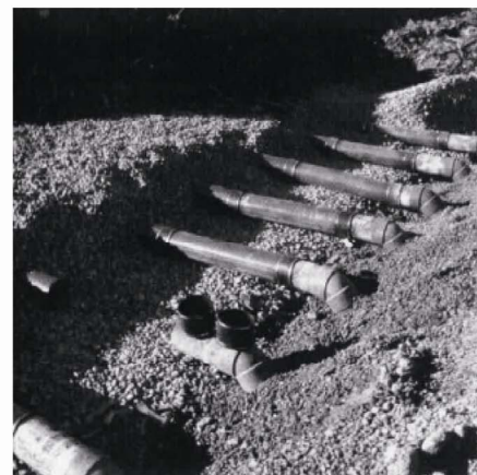
Figure 1. (Left): Schematic of a biofilter using compost and compost sieving and (Right): photograph of aerator pipes leading into a soil or compost biofilter [11].
